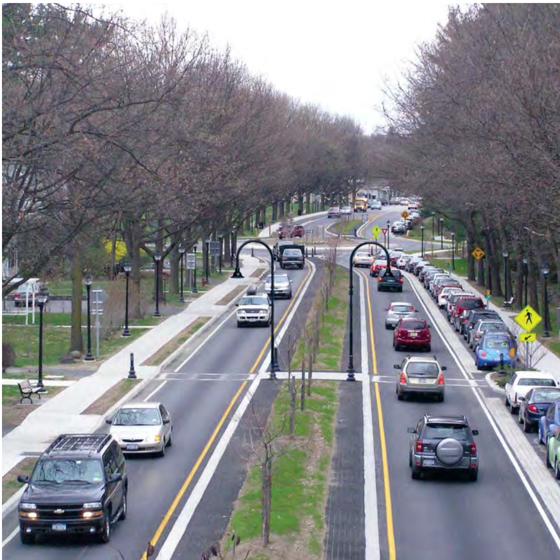
Figure 7-9. Divided Arterial Street with Parking Lane
