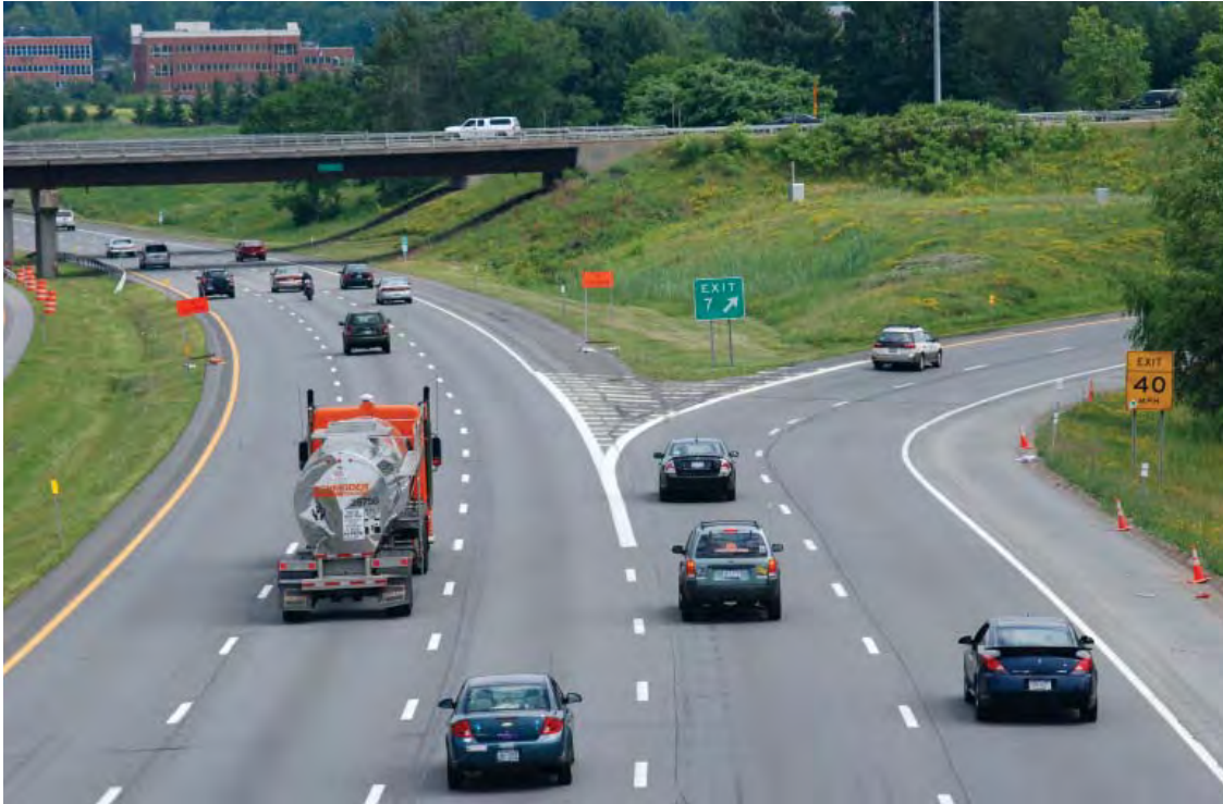
Figure 10-66. Gore Area, Two-Lane Exit
