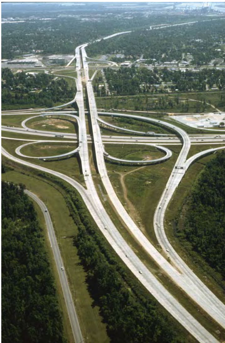
Figure 10-42. Cloverleaf Interchange with Semidirect Connection
