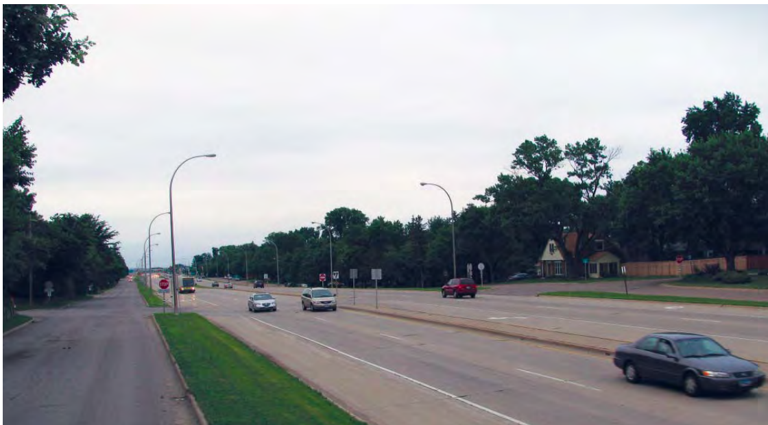
Figure 7-11. Divided Arterial Street with Two-Way Frontage Road
