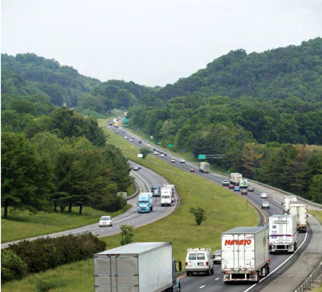
Figure 8-1. Typical Ground-Level Rural Freeway
