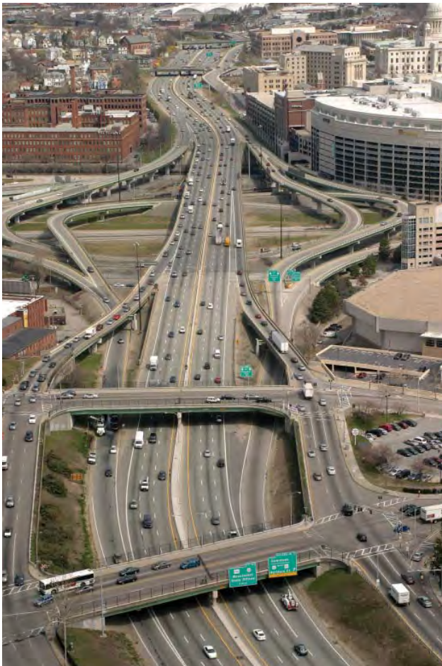
Figure 8-17. Combination-Type Freeway
