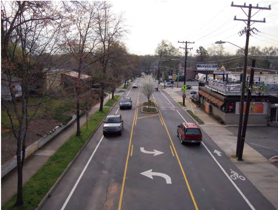
Figure 7-7. Continuous Two-Way Left-Turn Lane
