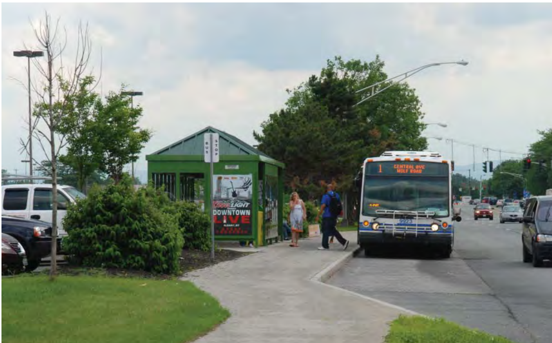
Figure 4-23. Midblock Bus Turnout
