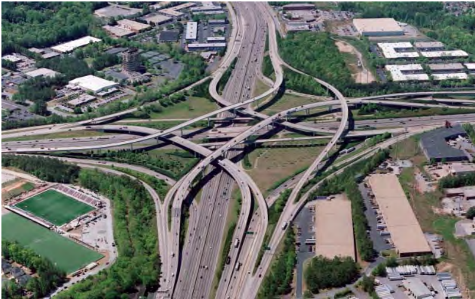
Figure 10-36. Four-Level Directional Interchange
