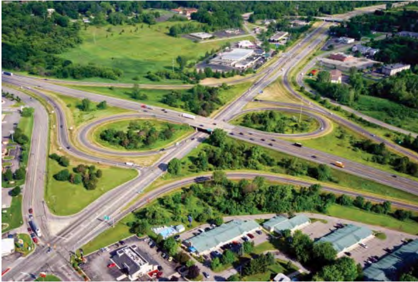
Figure 10-27. Partial Cloverleaf Interchange
