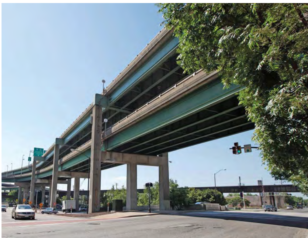
Figure 8-11. Two-Level Viaduct Freeway
