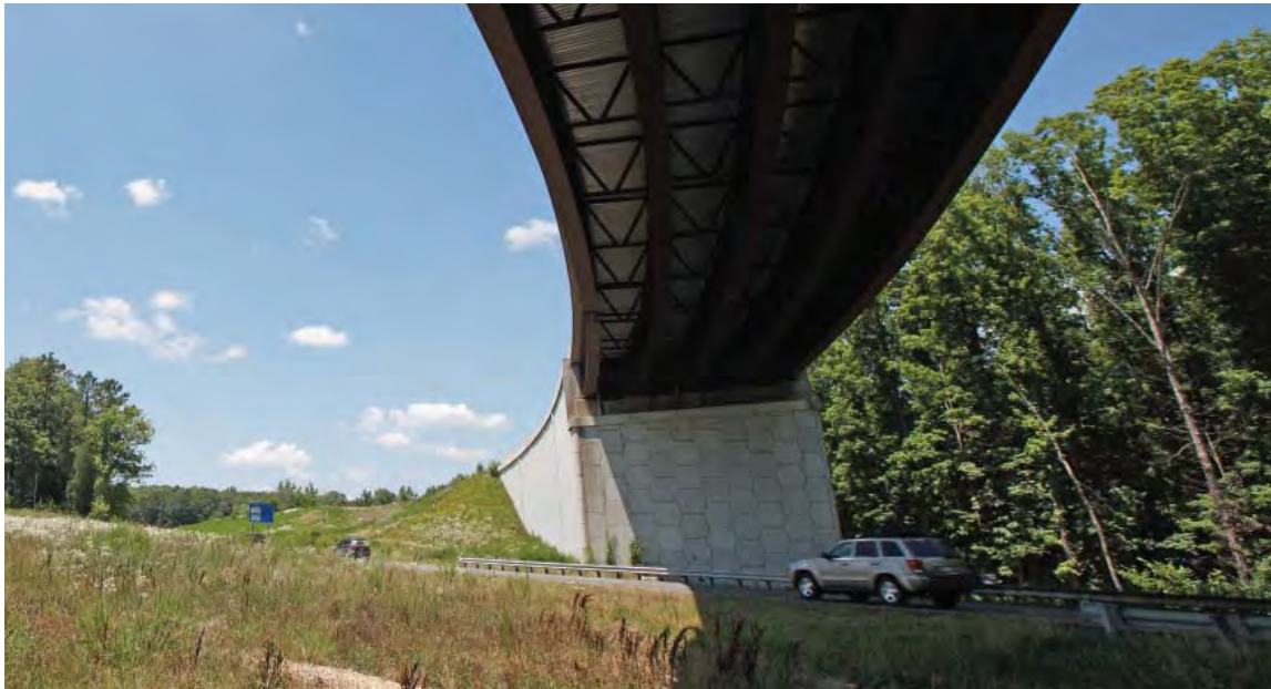
Figure 10-3a. Typical Grade Separation Structures with Closed Abutments
