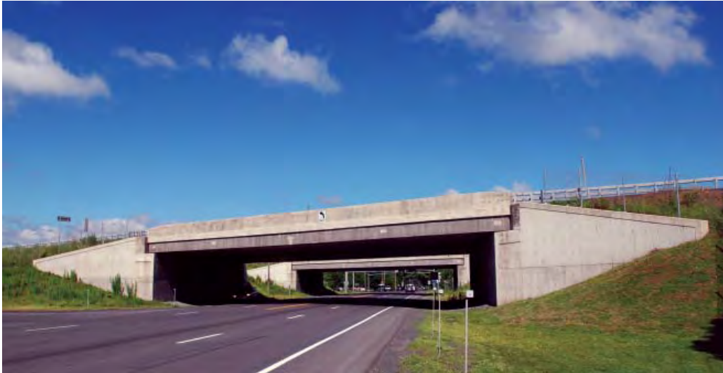
Figure 10-3b. Typical Grade Separation Structures with Closed Abutments
