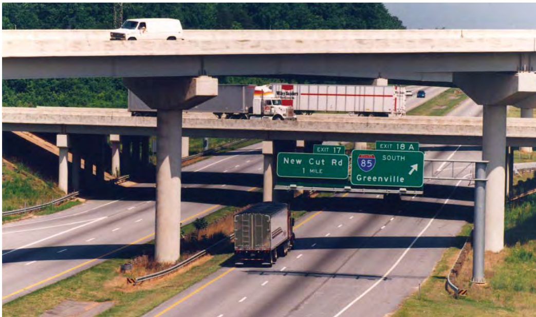
Figure 10-5. Multilevel Grade Separation Structures
