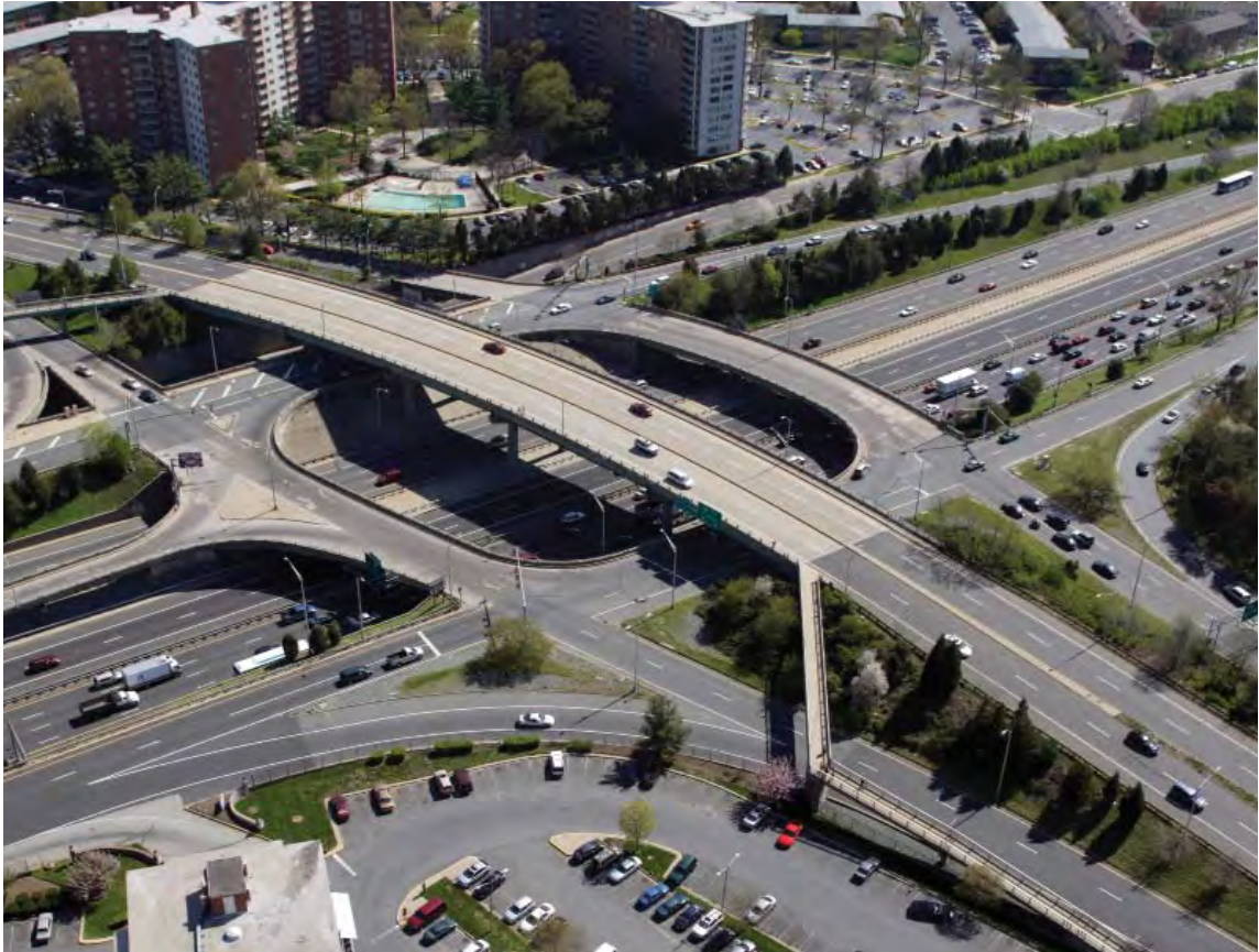
Figure 10-20. Freeway with a Three-Level Diamond Interchange
