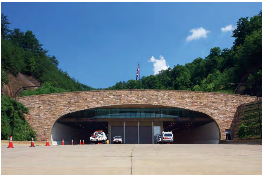
Figure 4-16. Entrance to a Freeway Tunnel
