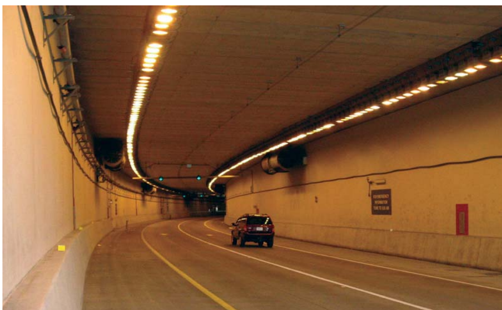
Figure 4-17. Interior of a Two-Lane Directional Tunnel
