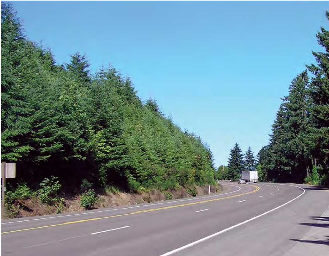
Figure 7-1. Climbing Lane on Two-Lane Rural Arterial
