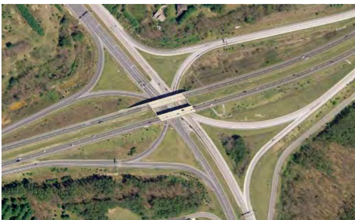
– B – Overpass SPDI
