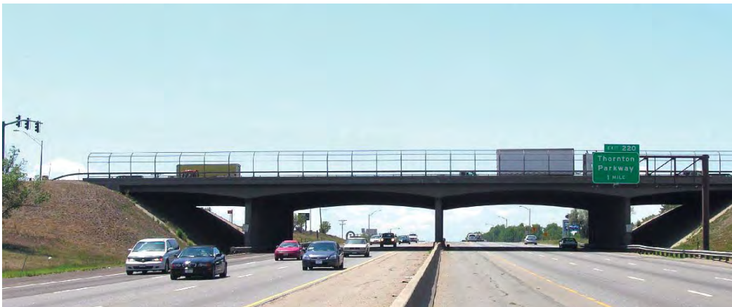
Figure 10-4. Typical Grade Separation Structure with Open-End Span
