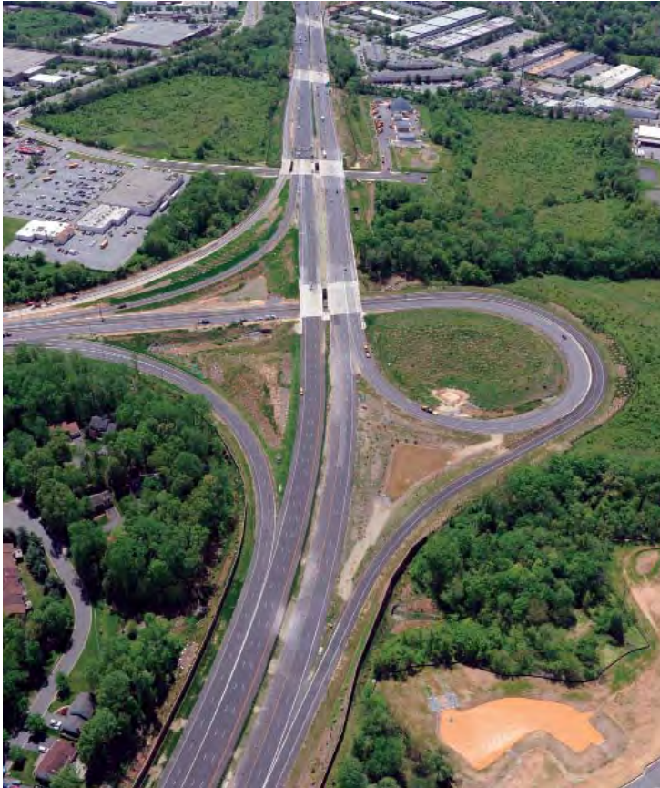
Figure 10-14. Trumpet Freeway-to-Freeway Interchange
