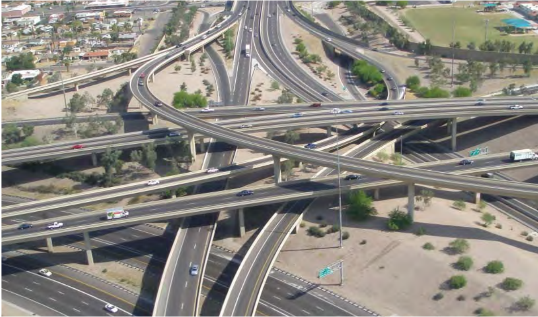
Figure 10-37. Four-Level Directional Interchange
