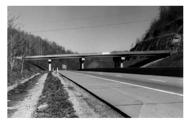
Exhibit 10-4. Typical Grade Separation Structure With Open-End Span
