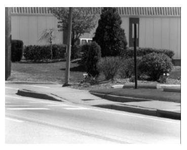
Exhibit 4-24. Sidewalk Curb Ramp at End of Curb Radius
